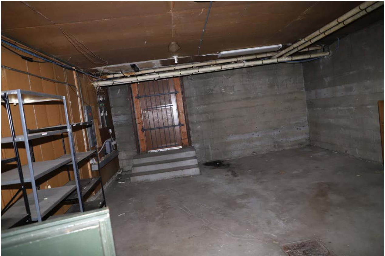
Photo 17. Basement, mechanical area and basement doorway, looking west.
