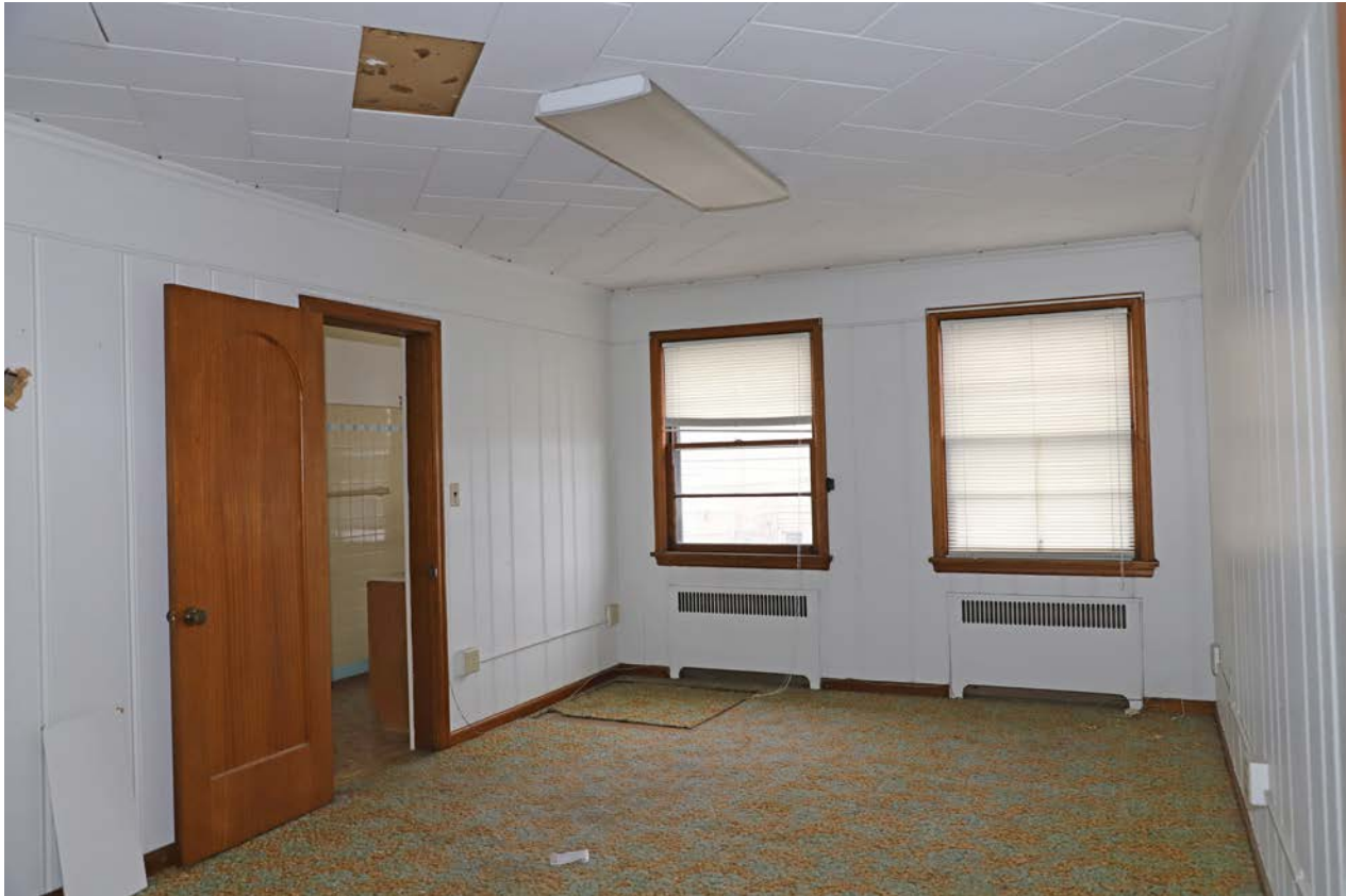
Photo 34. Second floor, bedroom, northwest, looking west.
