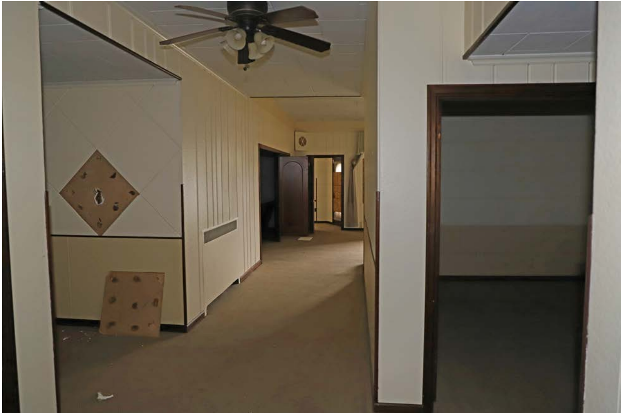
Photo 28. First floor, east/west corridor at north end of lobby, looking east.
