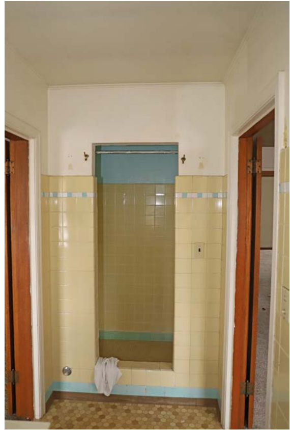
Photo 38. Second floor, north bathroom, looking east.
