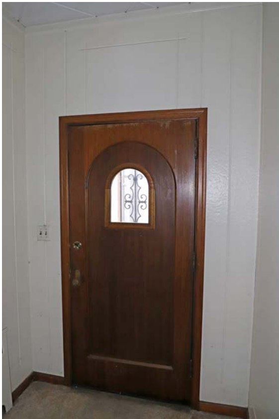
Photo 48. South stair, main entrance door for private residence.
