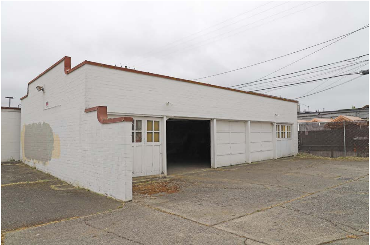
Photo 54. Garage, northeast corner.
