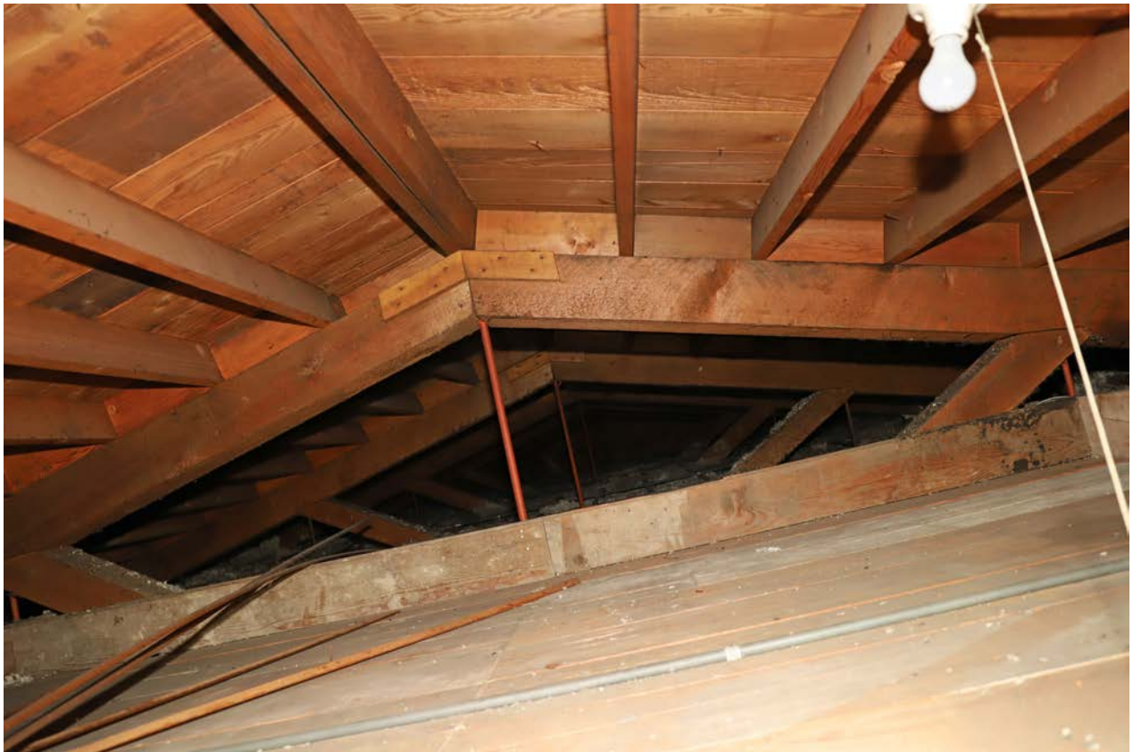
Photo 52. Second floor, attic space over north portion, looking north.
