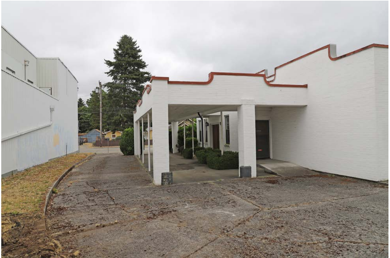
Photo 5. Exterior, northwest corner, looking east.
