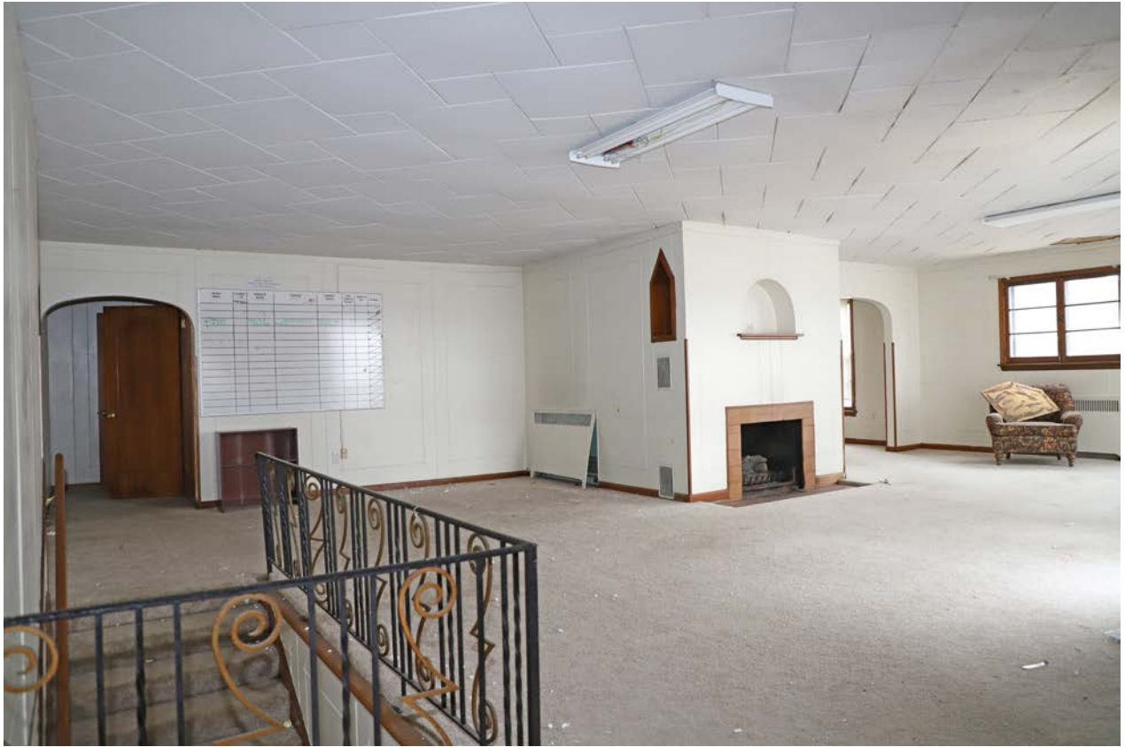
Photo 30. Second floor, living area, looking northeast.
