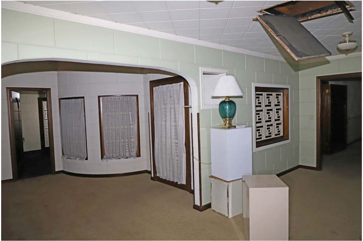
Photo 22. First floor, chapel, northwest corner looking east behind the dais.
