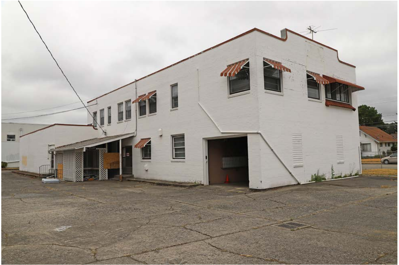
Photo 3. Exterior, southwest corner.
