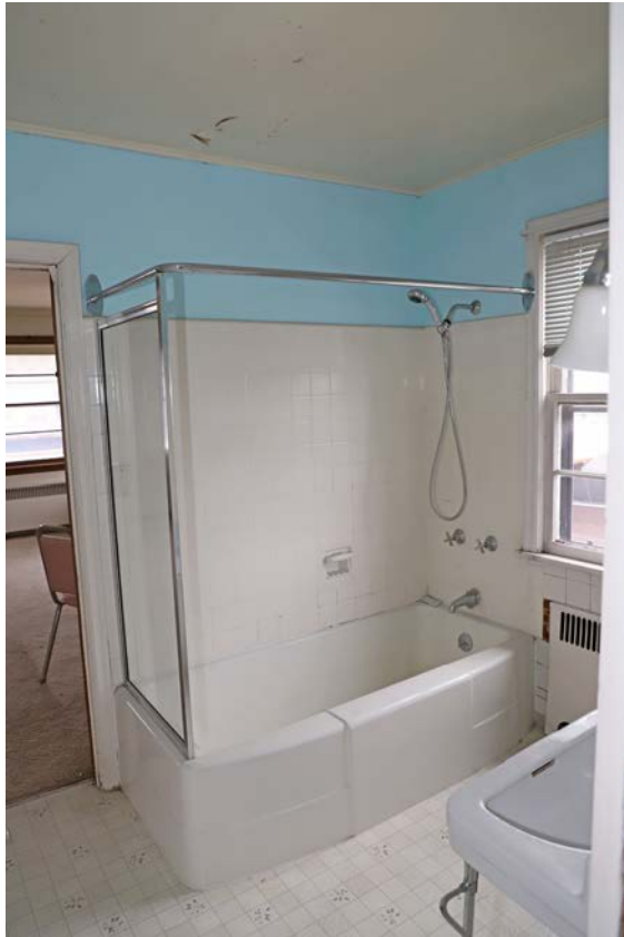
Photo 41. Second floor, bathroom, south, looking southwest.
