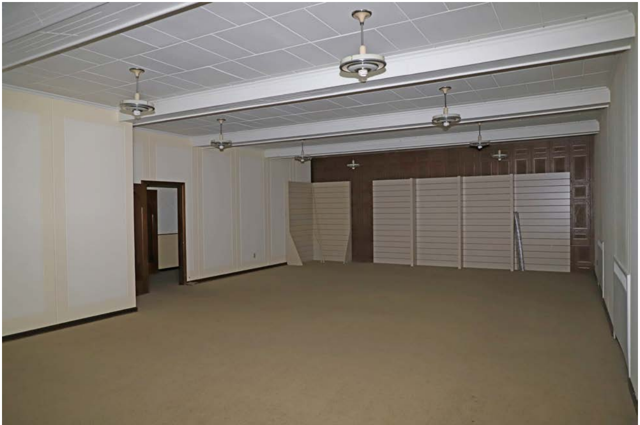
Photo 23. First floor, northwest volume, looking southeast.
