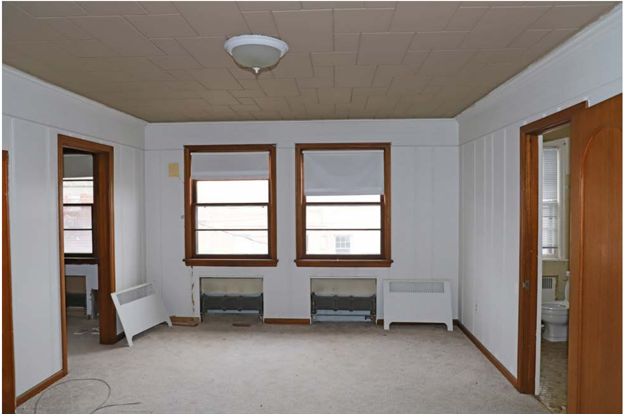
Photo 39. Second floor, bedroom, central, looking west.
