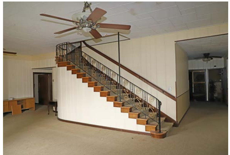
Central L-shaped stair, 2021.
