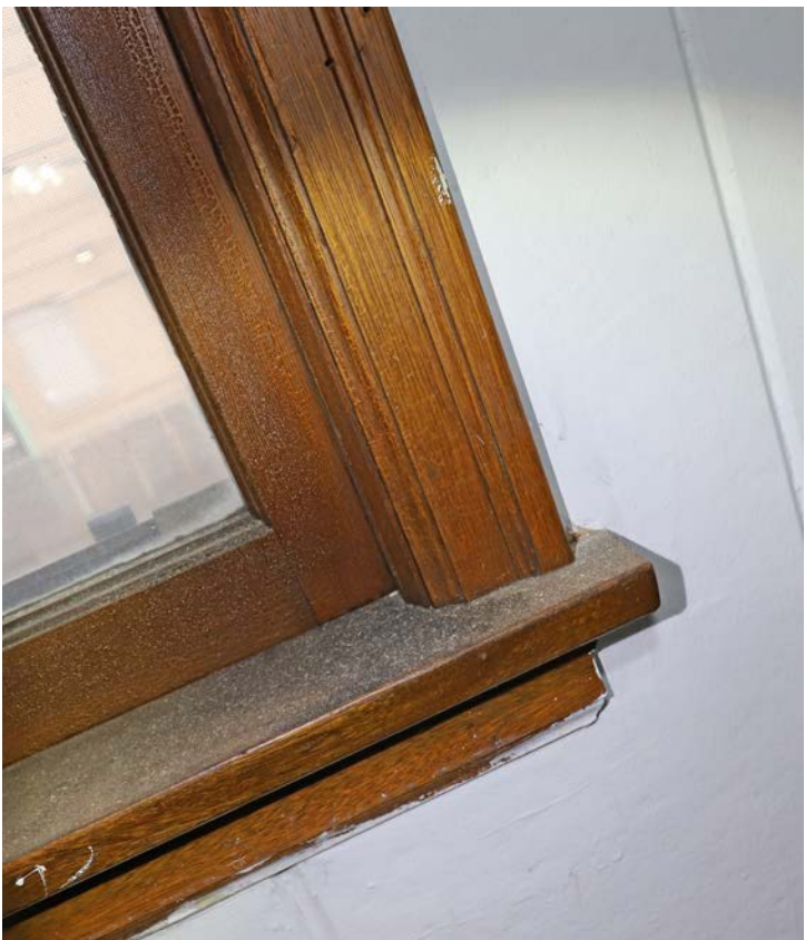
Photo 45. Second floor, casing detail.
