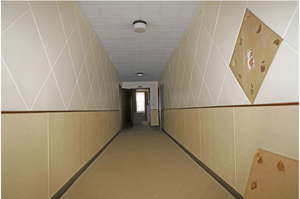
Photo 24. First floor, north/south corridor, looking north.
