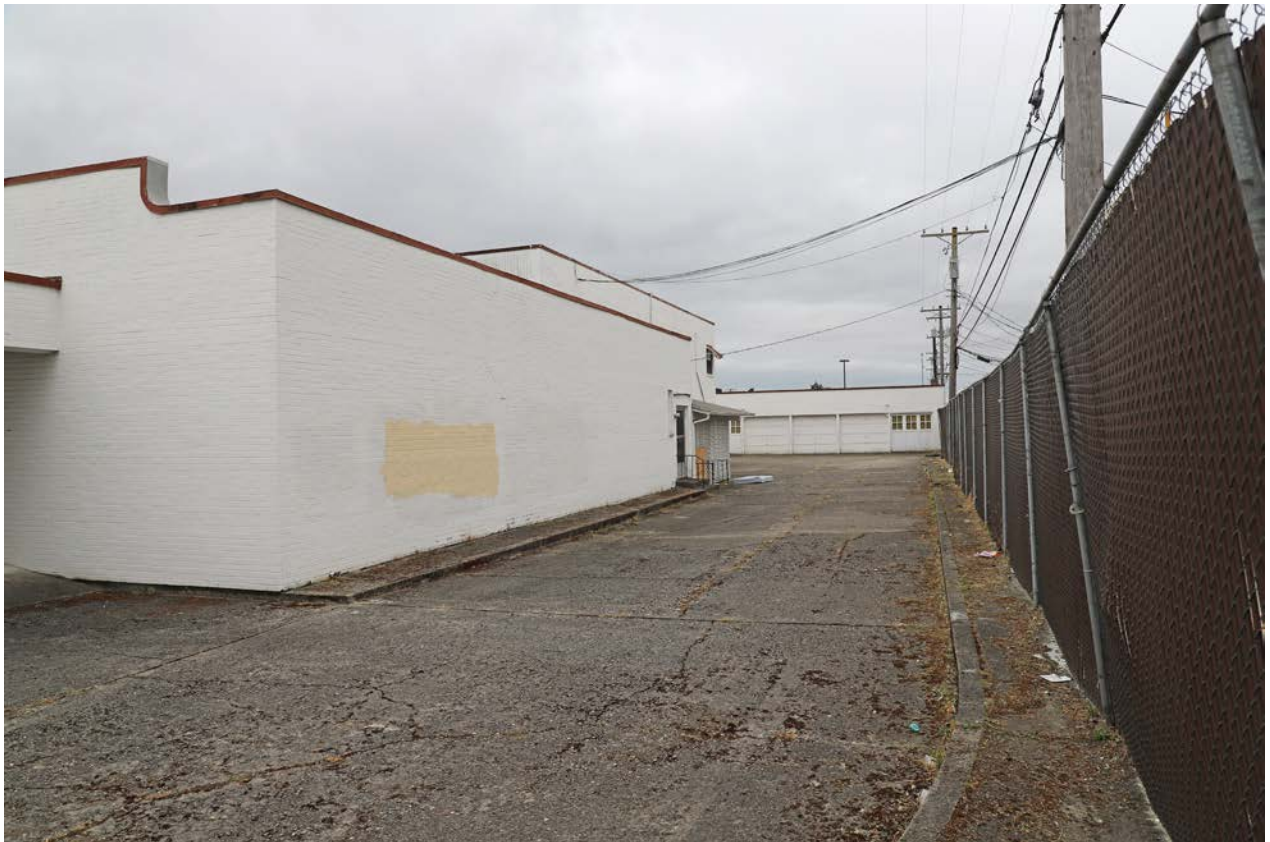
Photo 4. Exterior, northwest corner, looking south.
