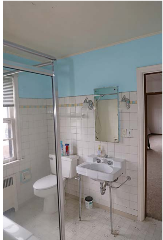
Photo 43. Second floor, bathroom, south, looking northwest.
