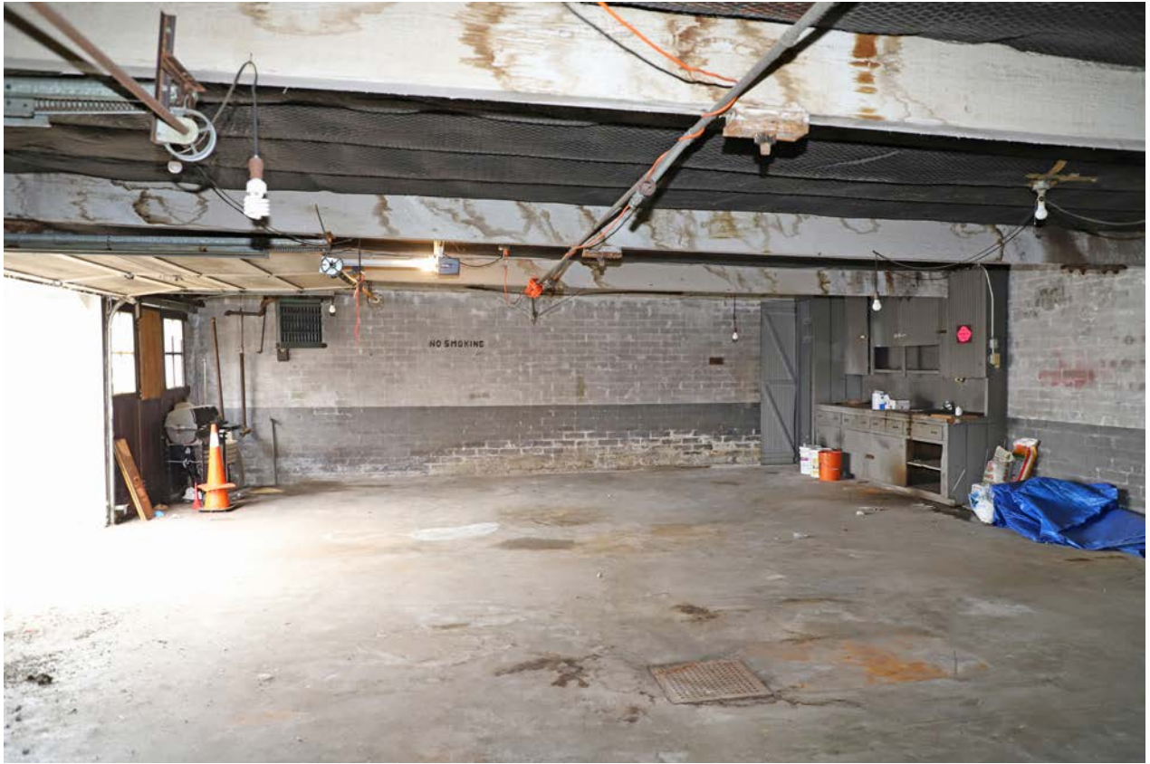
Photo 56. Garage, interior, looking east.
