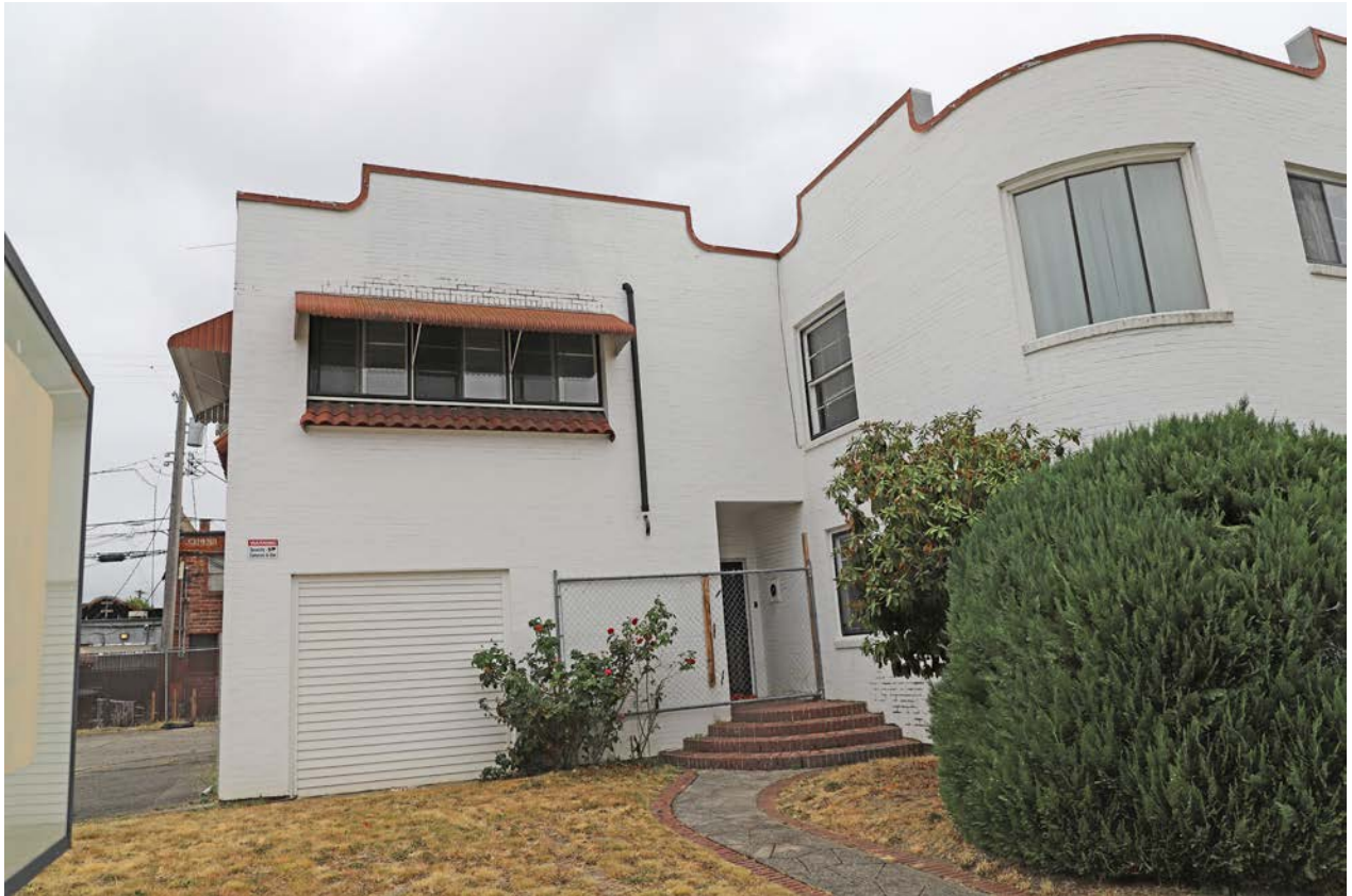
Photo 12. Entrances, southeast corner. Access to private residence and former garage door location.
