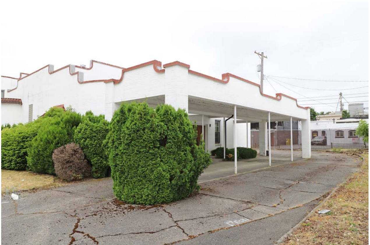
Photo 6. Exterior, northeast corner, looking southwest.
