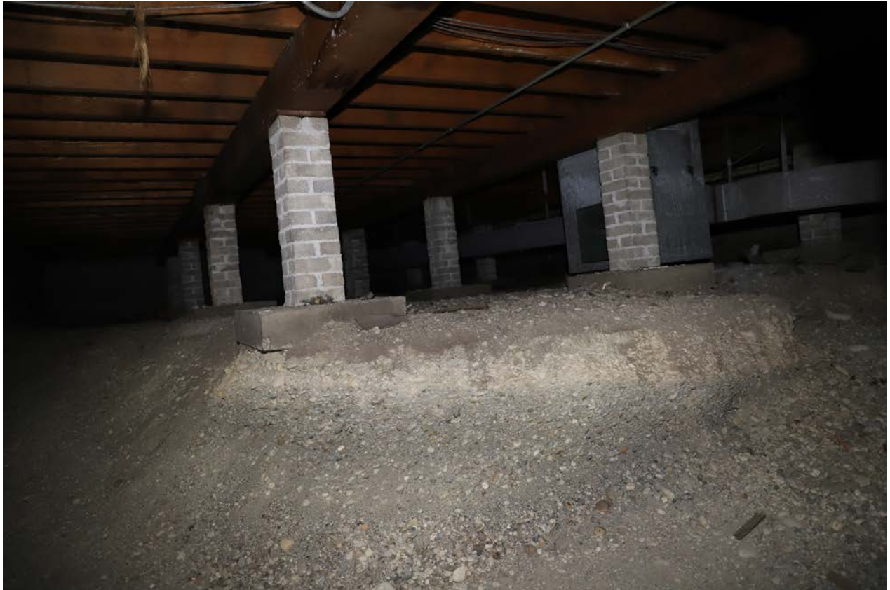
Photo 16. Basement, north end, crawl space.
