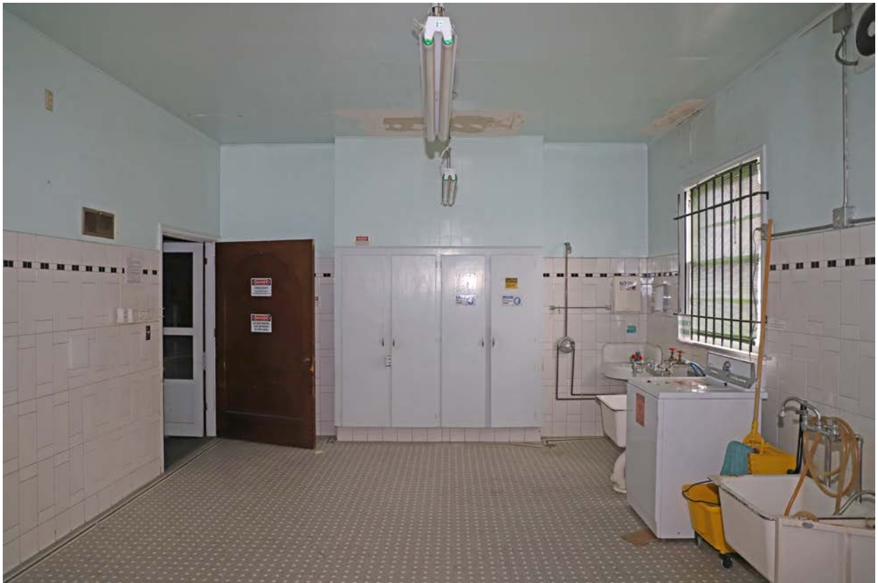
Photo 27. First floor, embalming space, looking south. The door at left opens to the receiving area.
