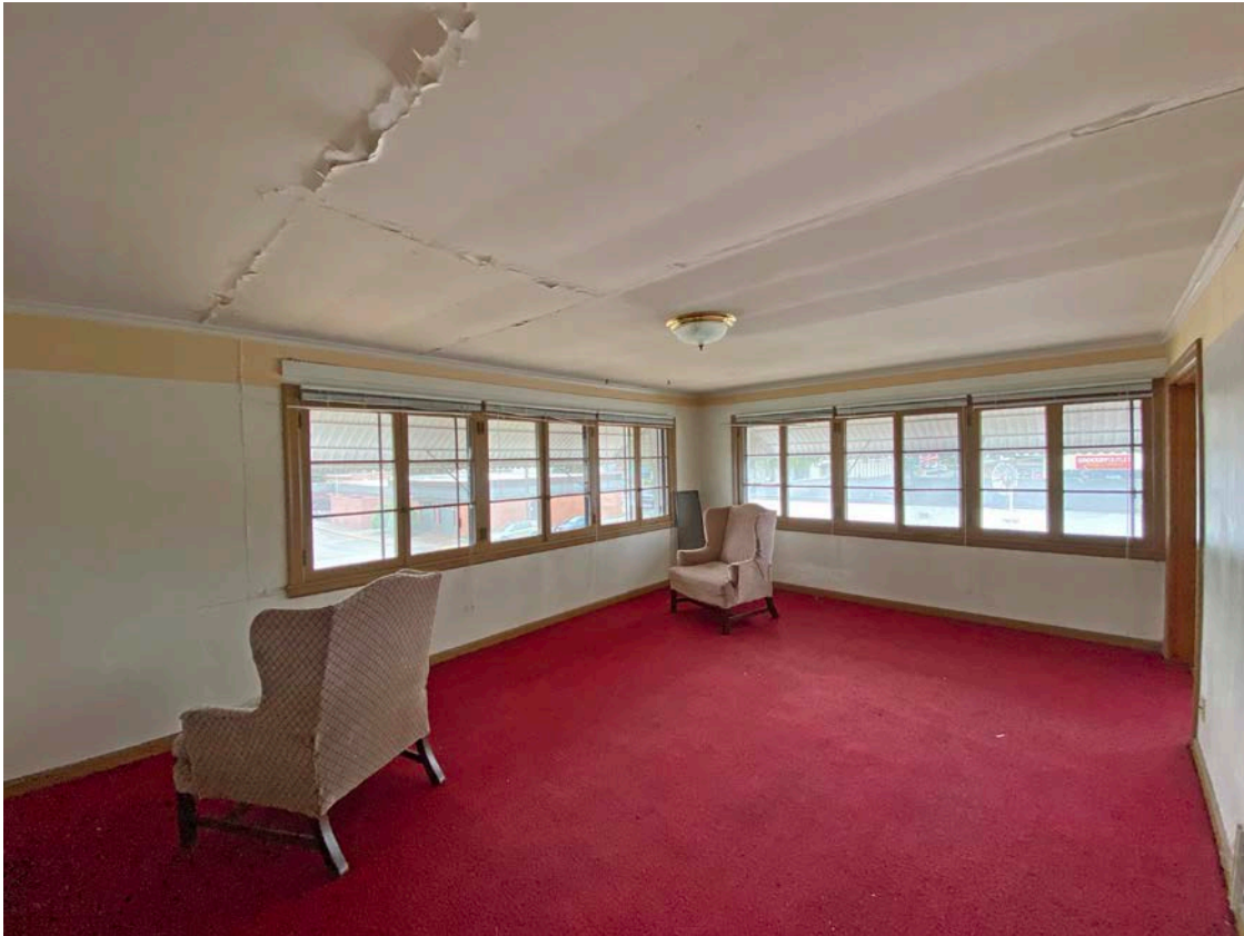
Photo 44. Second floor, sun room, looking southeast.
